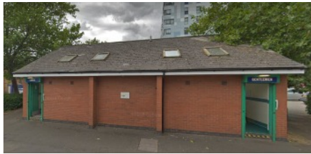
Albert Street Public Toilets
