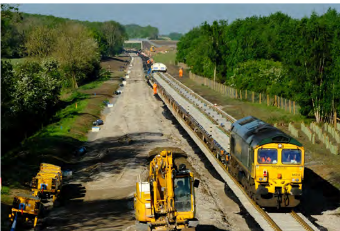
An engineering train on site
