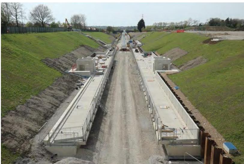
Winslow Station Platforms under construction in early May 2022
