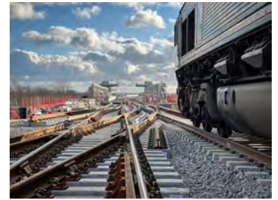
New track near Bletchley High Level Station
