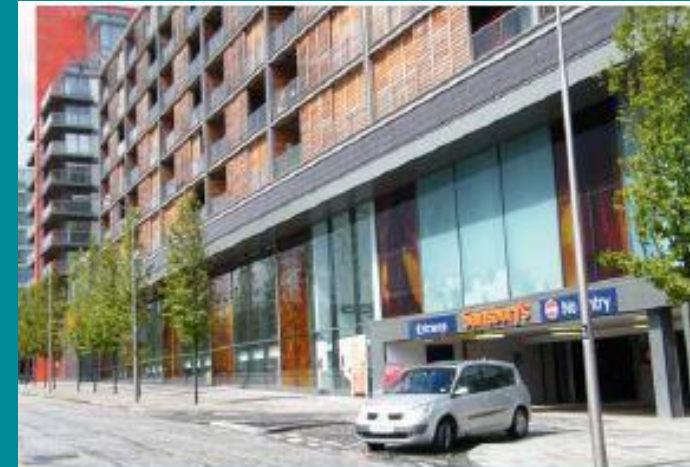
Integrated parking solution (Vizion Development, CMK) where the car park entrance is kept to a minimum and designed as part of building facade
